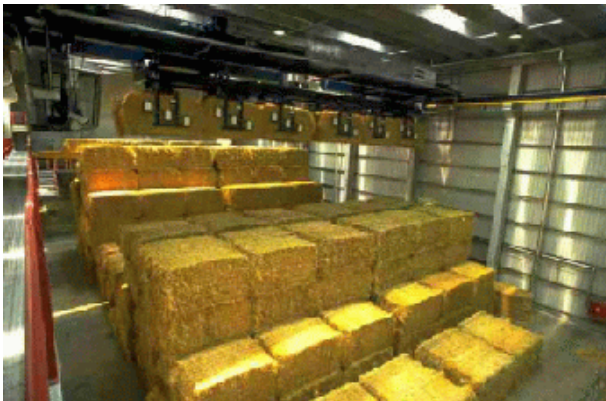
Figure 3: Straw unloading crane in operation
